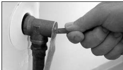
Figure 34 - Soupape DST
