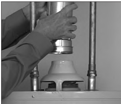
Figure 14 - Disconnect the vent pipe from the draft hood.
