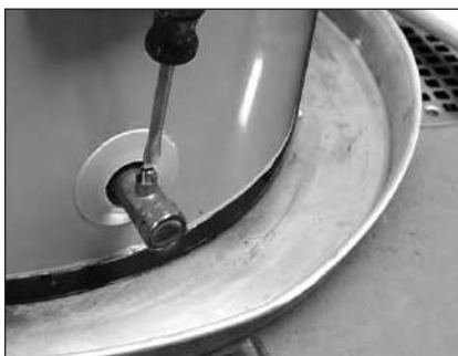
Figure 31 - Draining the water heater.
