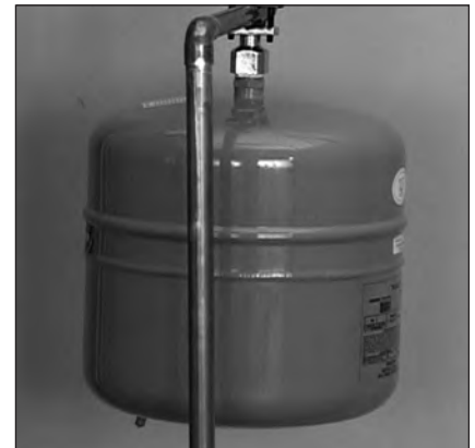
Figure 20 - The Thermal Expansion Tank should be pressurized with air to match the home's incoming water pressure.
