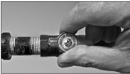
Figure 23 - Manual Gas Valve in ON position.
