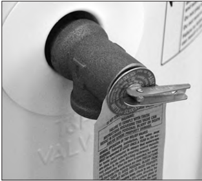
Figure 16 - Temperature and Pressure Relief Valve
