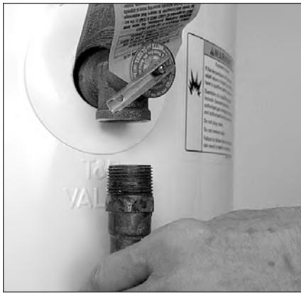
Figure 13 - Removing the T&P Relief Valve discharge pipe.
