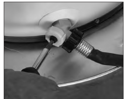
Figure 12 - Draining the old water heater.
