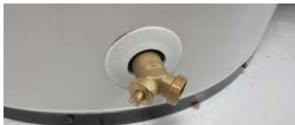
Figure 42 - Drain Valve
