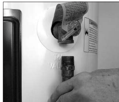
Figure 12 - Removing the T&P Relief Valve discharge pipe.
