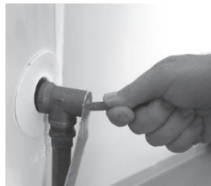
Figure 46 - T&P Relief Valve
