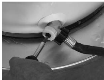
Figure 11 - Draining the old water heater.
