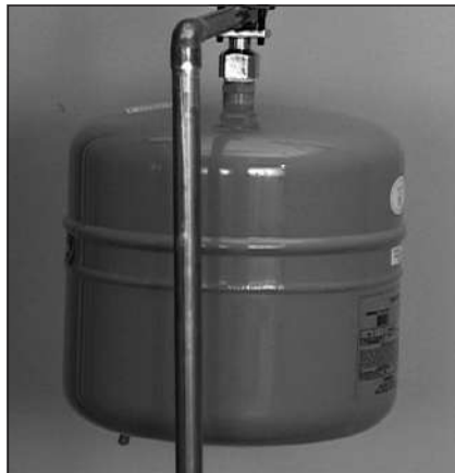
Figure 7 - A Thermal Expansion Tank helps protect the home's plumbing system from pressure spikes.
