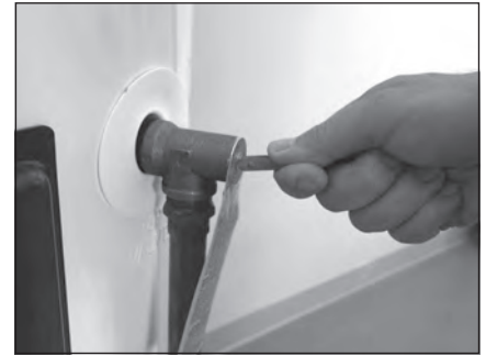
Figure 38 - Soupape DST.
