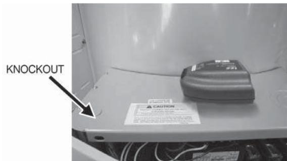
**Figure 32. Knockout on Left Corner of Top Panel**
