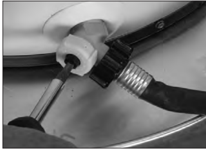
Figure 10 - Draining the old water heater.
