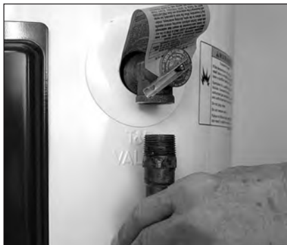
Figure 11 - Removing the T&P Relief Valve discharge pipe.
