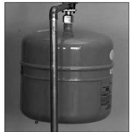
Figure 5 - A Thermal Expansion Tank helps protect the plumbing system from pressure spikes.
