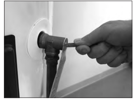
Figure 38 - T&P Relief Valve
