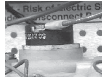
Figure 11. Éléments chauffants installés
