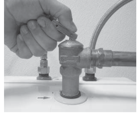
Figure 31 - T&P Relief Valve
