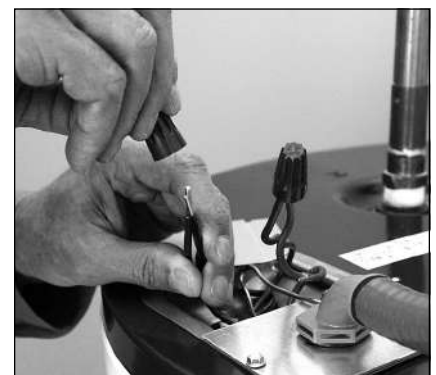
Figure 19 - Connecting the electrical wires.
