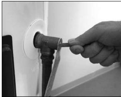
Figure 38 - T&P Relief Valve
